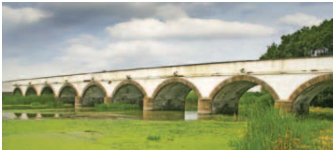
The Nine-holed Bridge
